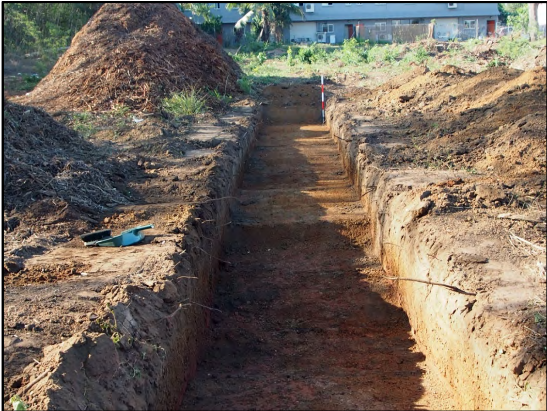
Figure 18: Trench 5 looking north showing shallow sands overlying yellow clays
